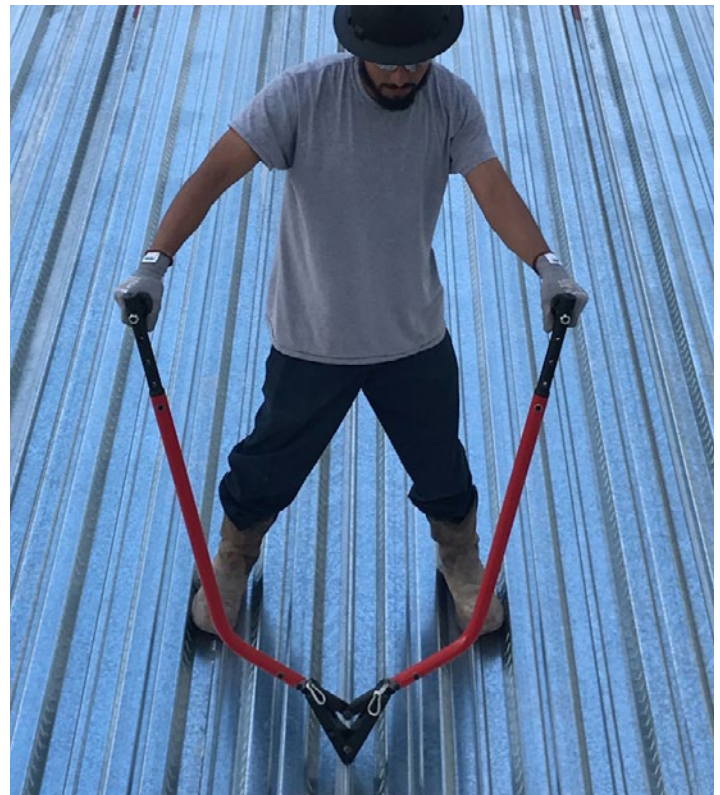
A typical steel deck installation
